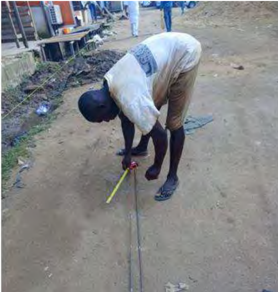
(Bethel Street ongoing reconstruction at Itire Ikate LCDA )
